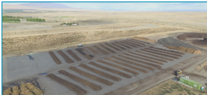
Horn Rapids Landfill composting facility.
