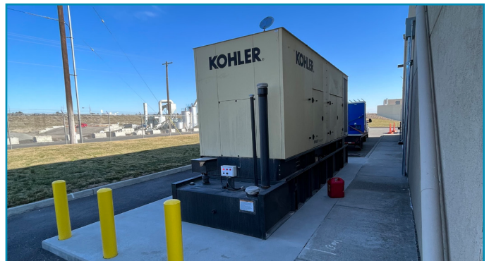
RH2 recently completed projects with the City that replaced the Digester Control Building motor control and HVAC equipment, and emergency generator at the Solids Handling Building.
