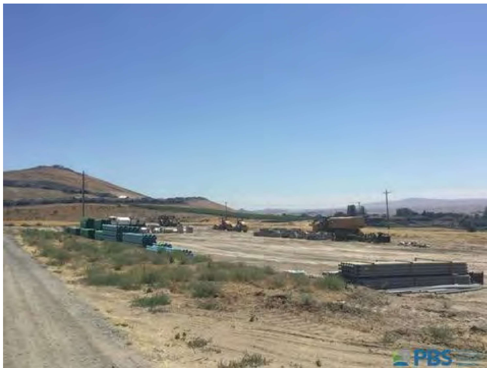
Photo 11. Southern adjacent property.
