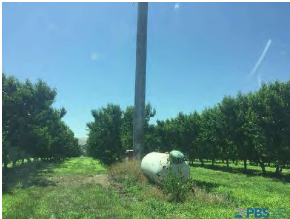
Photo 15. Empty ast and turbine.
