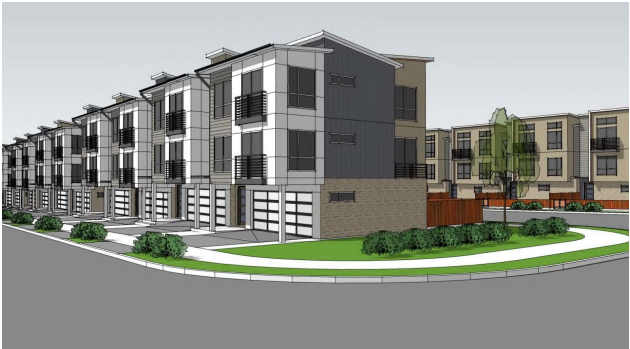
BLOCK CORNER VIEW
