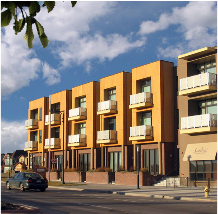
Illustrative Photo: Urban Character Live/Work Building
