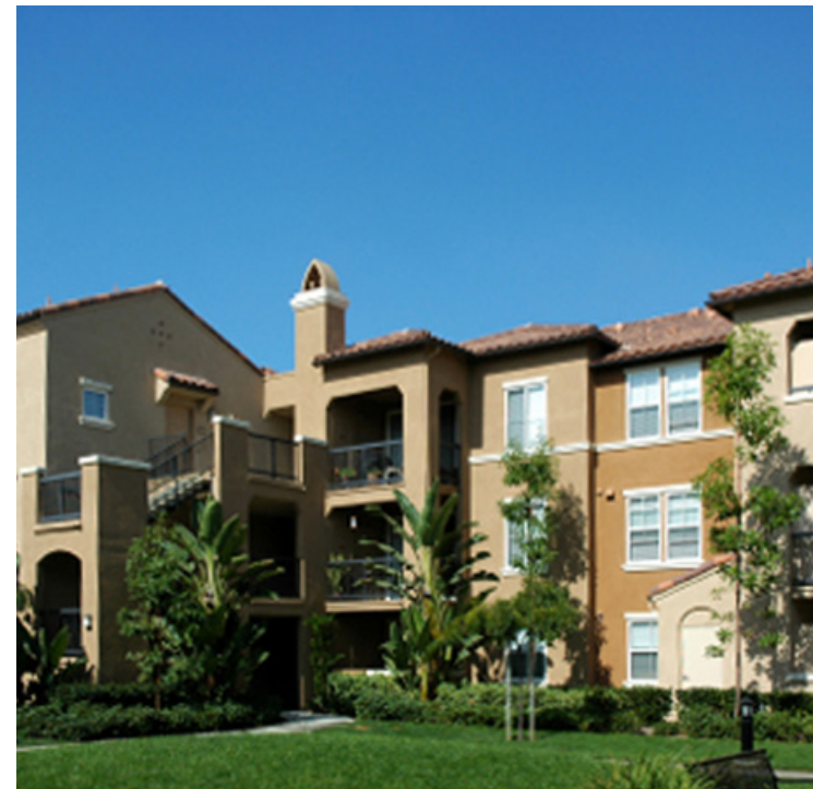
Illustrative Photo: Traditional Walk-up Apartment Building
