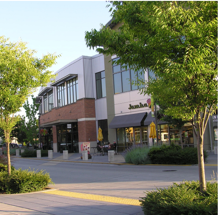
Illustrative Photo: Office above Retail Streetscape
