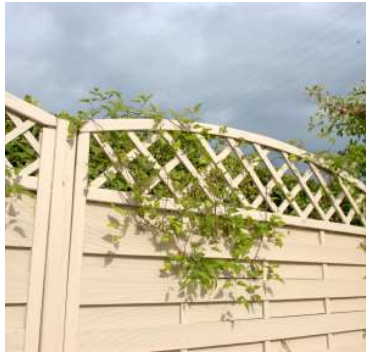
Side and Rear Yard Fencing
