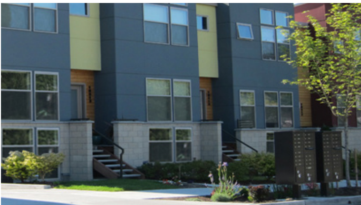
Illustrative Photo: Row House Stoop Frontages
