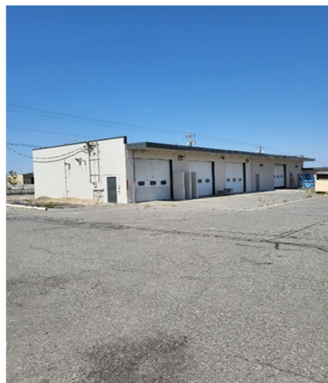
Figure 8-1. Benton County MRW Facility
