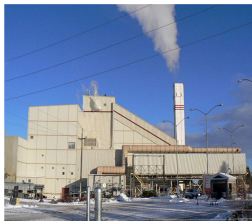
Figure 9-1. City of Spokane Waste-to-Energy Plant
