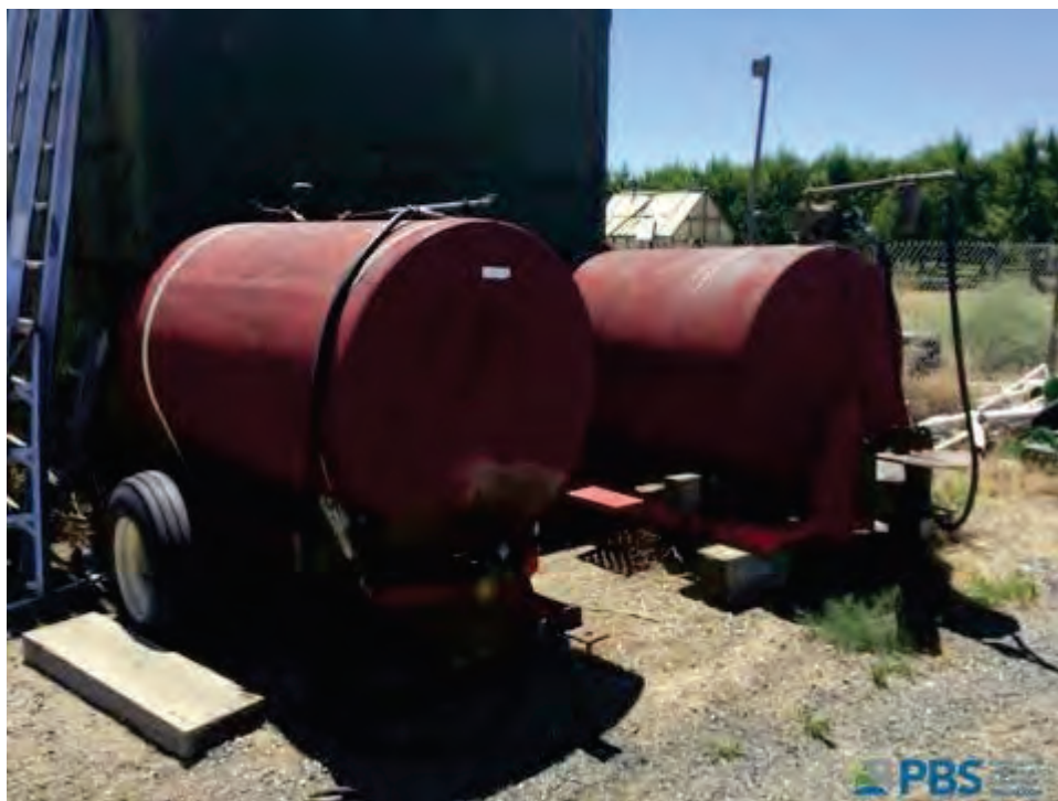
Photo 40. Mobile ast gasoline tanks.
