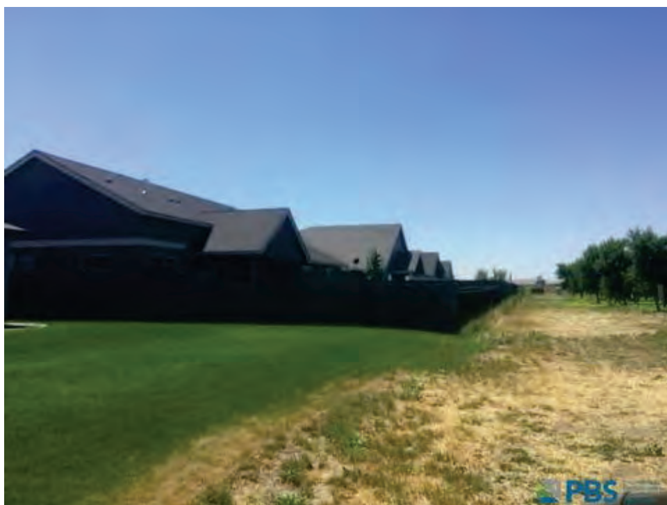
Photo 24. Adjacent residential houses.
