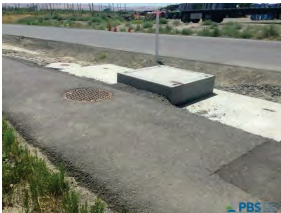
Photo 26. Utility access manholes.
