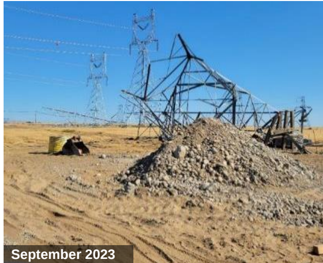
Demolition of aging electrical utility towers as part of the Bonneville Power Administration's North Loop Replacement Project
