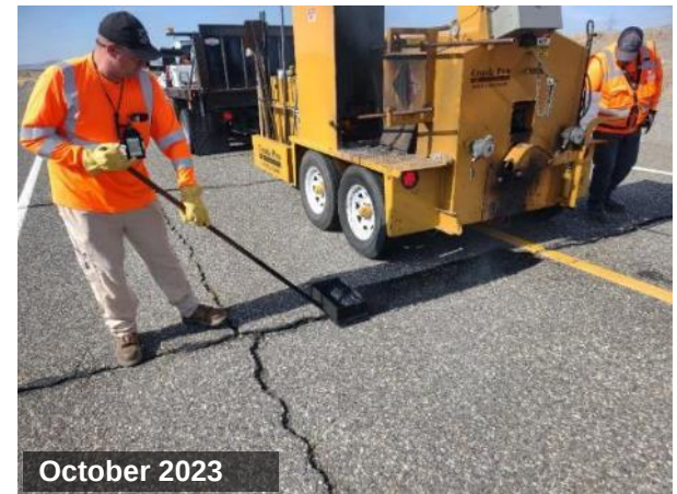
Repairs to State Route 10
