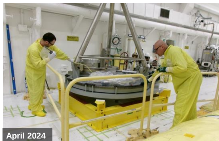
Workers install components for a transfer system at the Waster Encapsulation and Storage Facility
