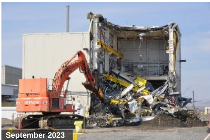
K West Annex Building demolition
