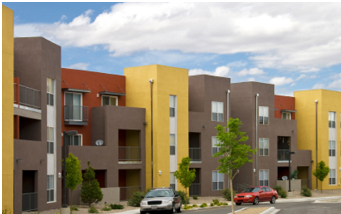
Stacked Unit Building (Apartment) (8H)
