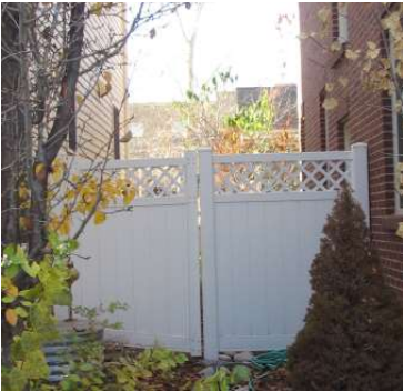
Wing-Fencing with Gate
