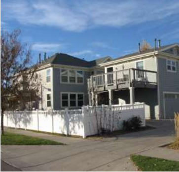
Corner Lot Fencing
