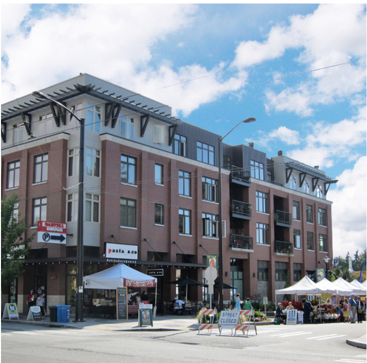
Illustrative Photo: Residential Units above Retail Frontage
