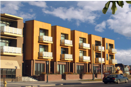
Live/Work Building (8G)
