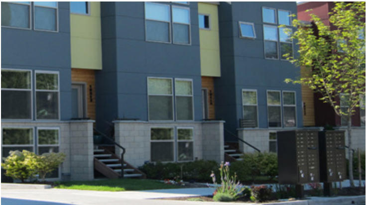
Illustrative Photo: Row House Stoop Frontages
