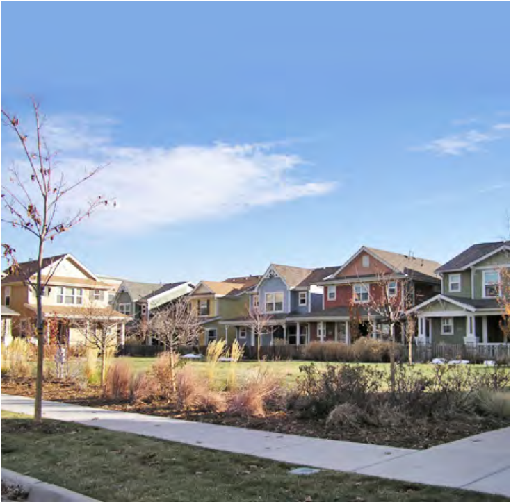
Illustrative Photo: Corner Block Cottage Court
