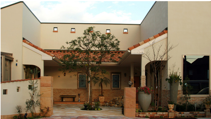
Illustrative Photo: Residential Entry Court
