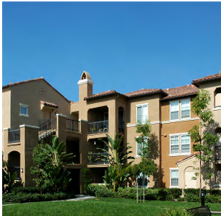
Illustrative Photo: Traditional Walk-up Apartment Building
