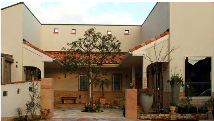
Illustrative Photo: Residential Entry Court
