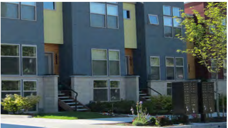
Illustrative Photo: Row House Stoop Frontages
