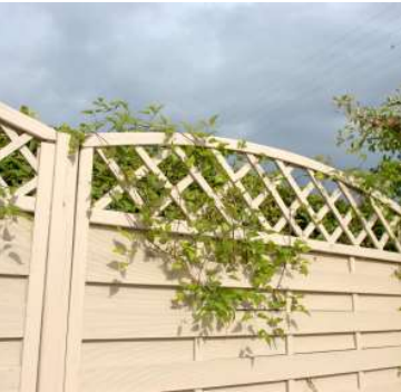
Side and Rear Yard Fencing
