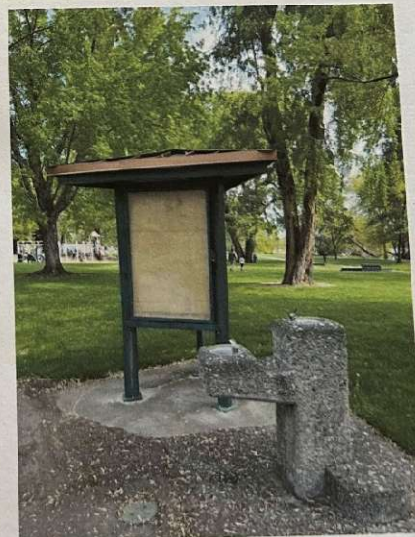
Figure 2B. Existing kiosk located in vicinity of Park Street playground
