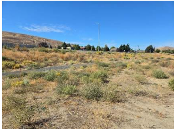
Photo Point Location 7. Southwest-facing view at the Keene Road embankment, showing the retention pond facility access road.
