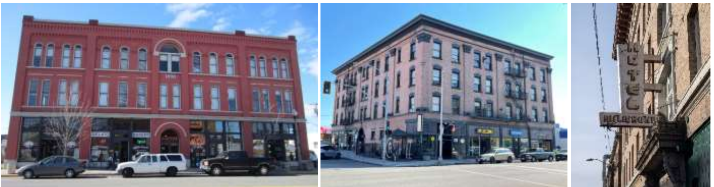
Left. The historic Wilson Hotel building, built 1890, is now managed by the Anacortes Housing Authority and functions as co-living housing with ground floor commercial businesses (source: MAKERS). Middle: The Upton Hotel in Spokane, built in 1910 and now known as the Grand Coulee Apartments, is listed on the National Register of Historic Places (Source: Will Maupin, CC BY-SA 4.0 ). Right. Milwaukee Hotel is one of several SROs still in operation in Seattle's Chinatown International District neighborhood. (Source: MAKERS)
