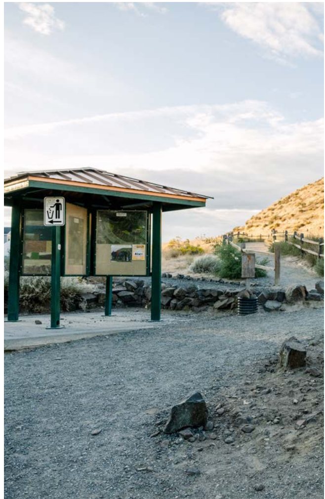
Kiosk at Badger Flats Trail
