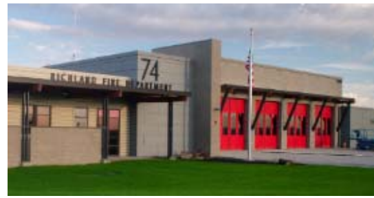
Richland Fire Station 74
