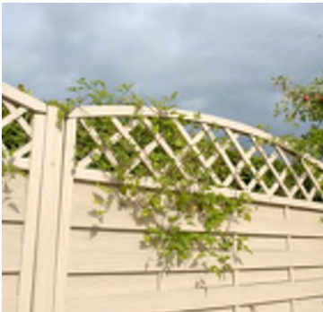
Side and Rear Yard Fencing
