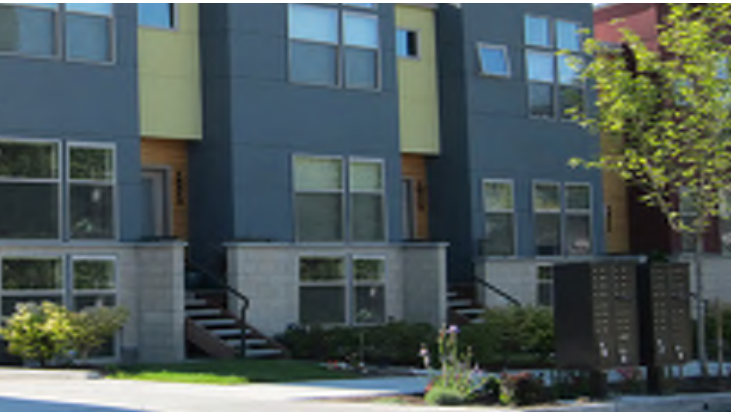
Illustrative Photo: Row House Stoop Frontages
