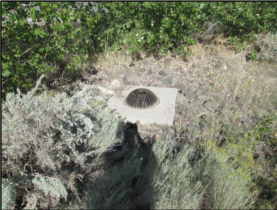
Photo 4: This photo shows a storm drain within the Preserve. This drain outlets stormwater stemming from the residential developments immediately west of the Preserve.
