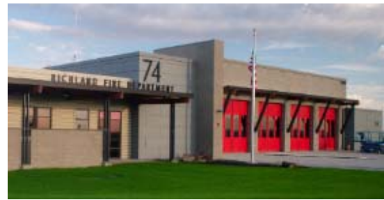
Richland Fire Station 74
