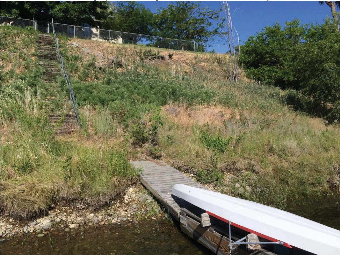
Photograph 4. Existing shoreline conditions at the project site; upriver of the proposed project.
