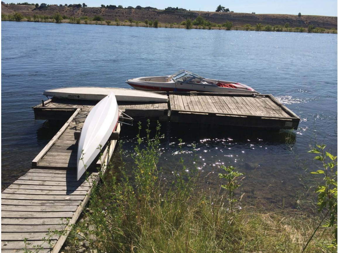
Photograph 6. Existing dock to be removed and replaced.
