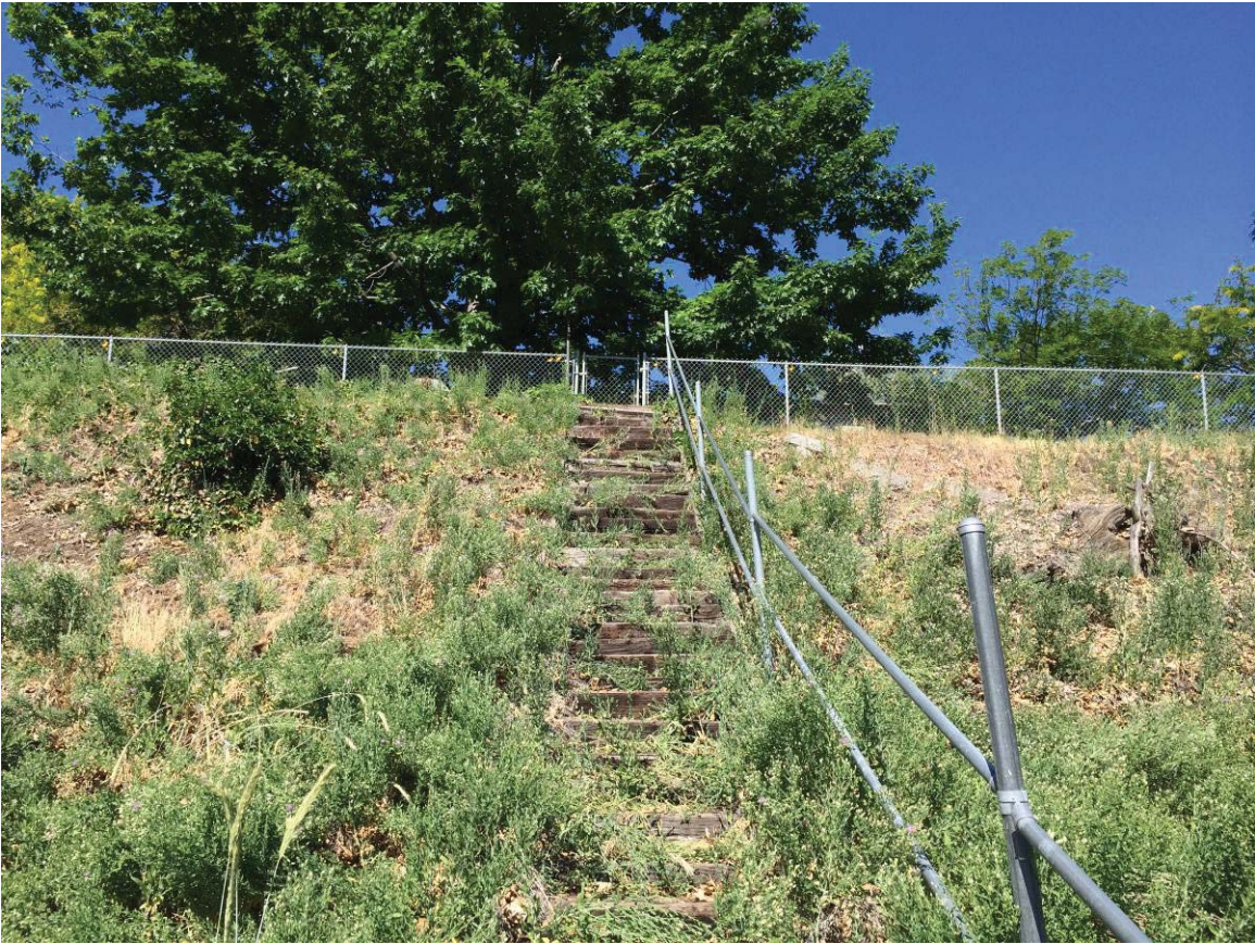
Photograph 3. Existing stairs to be removed and replaced.
