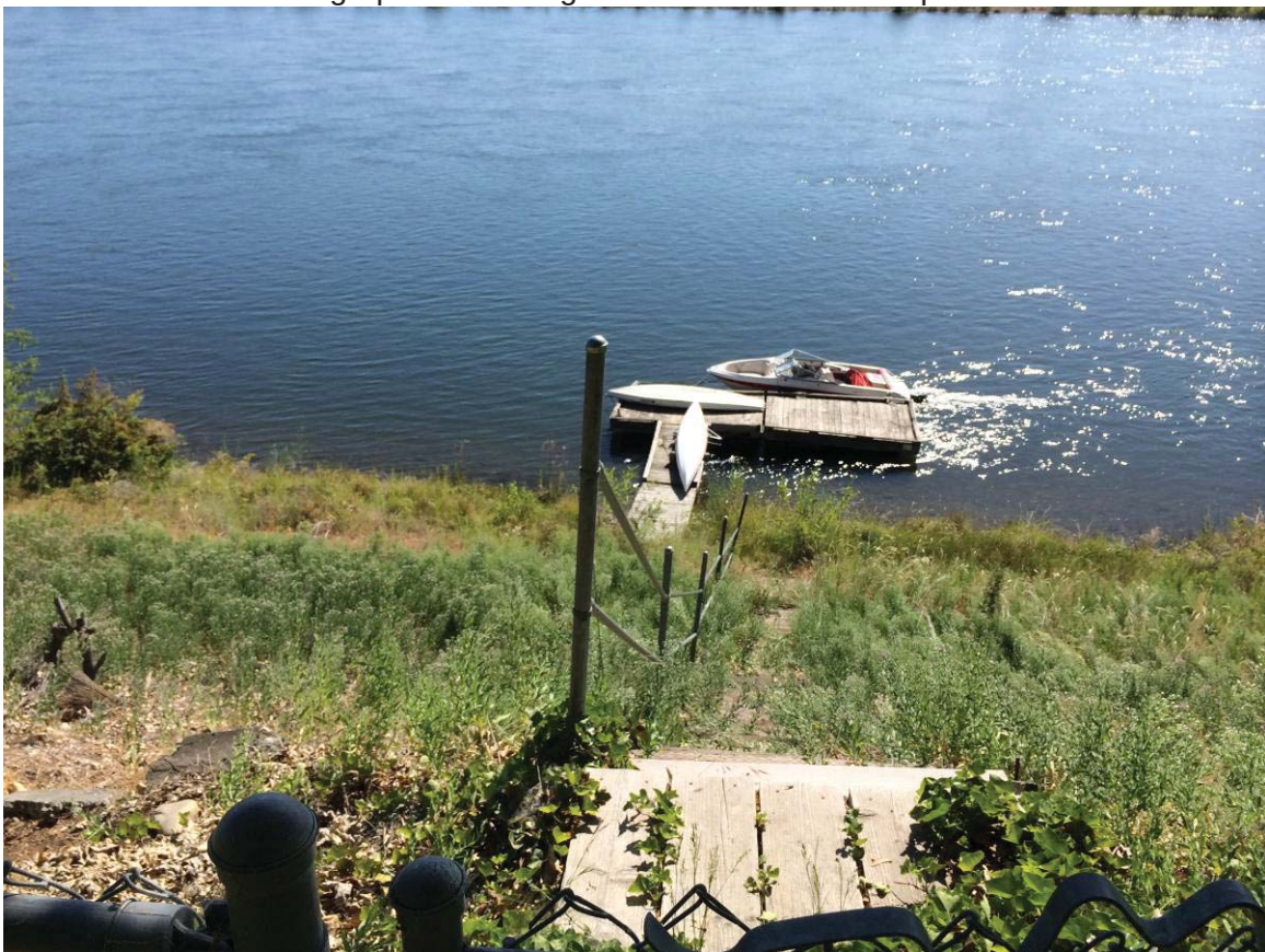
Photograph 2. Existing dock and stairs to be replaced.
