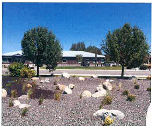
The Arc of Tri-Cities Parking Lot Expansion
