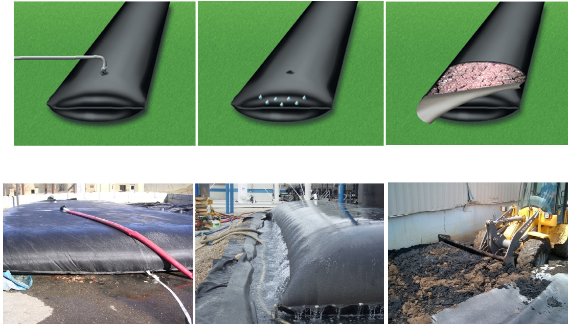
FIGURE 6 Typical Geotube Operation
