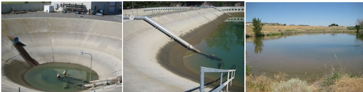
FIGURE 1 Richland WTP Solids Handling: Equalizing Basin, Sedimentation Basin, and Evaporation Pond
