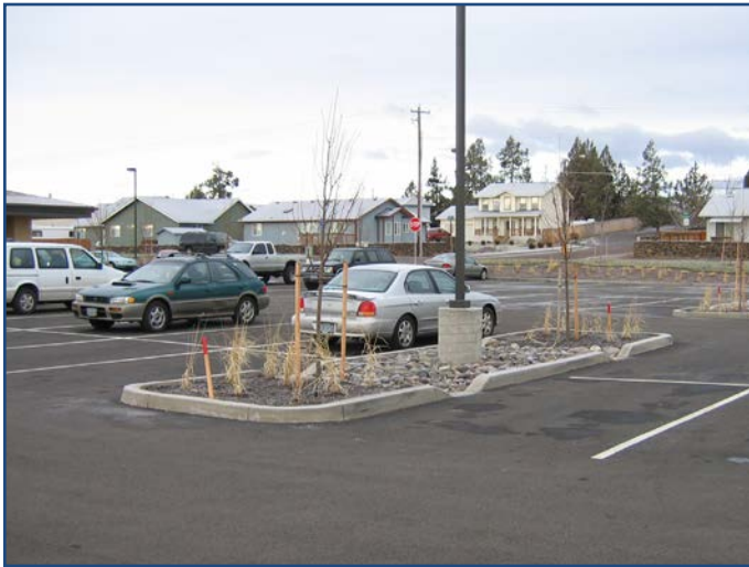
Example xeriscaped parking lot bioretention swales.
