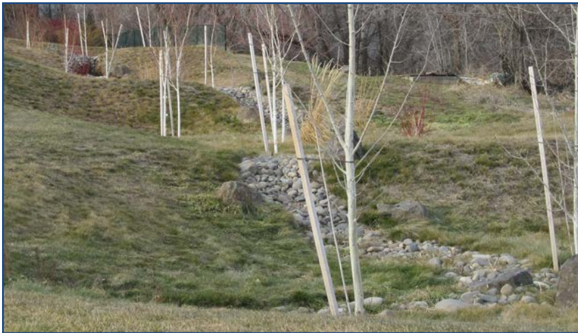
Example of cascading bioretention swales.
