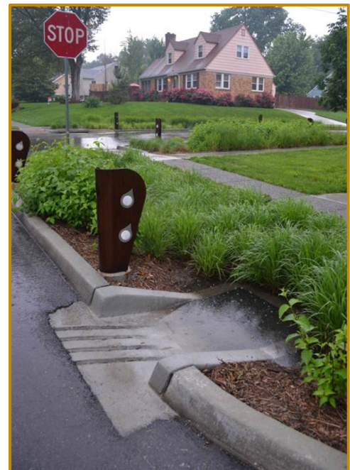
Example photo of a curb cut inlet into a bioretention facility (not the preferred approach.)
