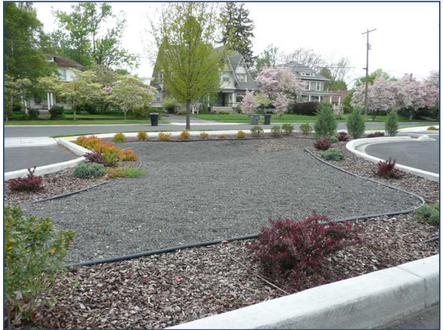
Example bioretention swale with a xeriscaped approach. Lower zone comprised of pea gravel and upper zone comprised of select grasses, shrubs, and trees.
