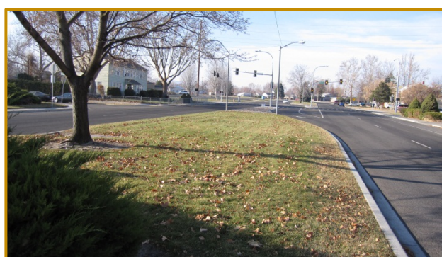
Swift Blvd. Median Looking West
