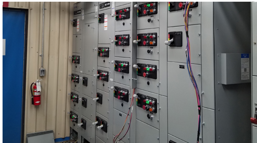
Headworks MCC replacement while under operation
