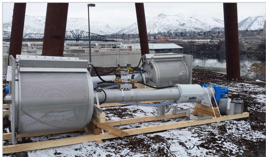
Headworks screen prior to construction
