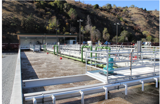
RH2 assisted the City of Cashmere with one of its biggest endeavors by providing comprehensive engineering services to complete their new 1.1 MGD WWTF.
