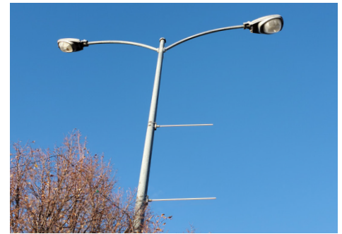
High Pressure Sodium light fixtures on George Washington Way, north of Williams Boulevard
