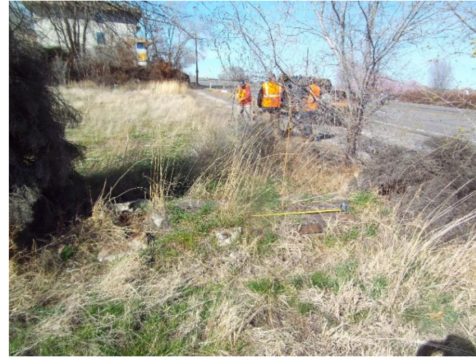
Figure 18. Closer view of basalt and mortar structure looking northwest. Tape measure is at one meter in length.
