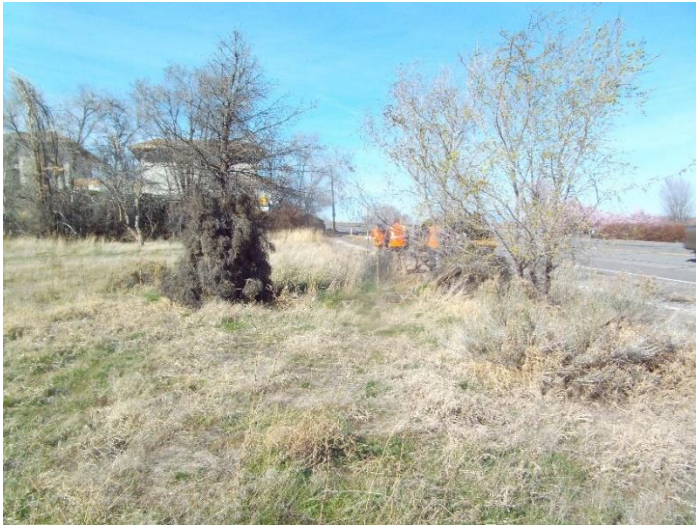
Figure 17. Overview of basalt and mortar structure located in grass looking northwest. Note the bushes to each side.
