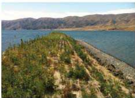
Armored and Planted Jetty and Shoreline
