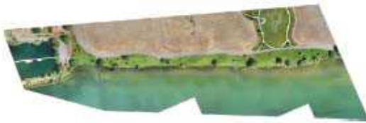
High resolution Columbia River Shoreline aerial captured by MacKay Sposito UAV
