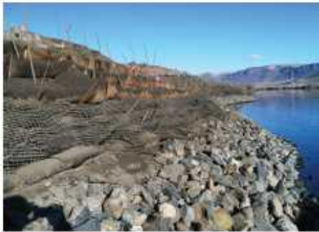
Bio-engineered and armored shoreline stabilization, Columbia River
