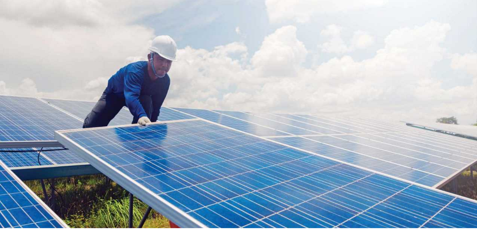
Engineer installing solar panel.
