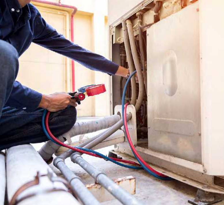
Technician measuring air conditioning equipment.
