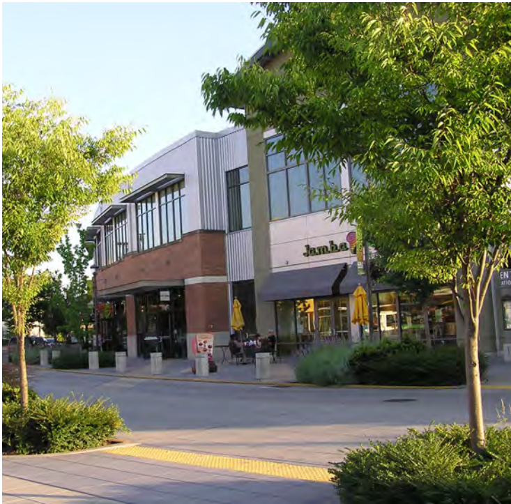
Illustrative Photo: Office above Retail Streetscape
