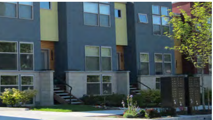
Illustrative Photo: Row House Stoop Frontages
