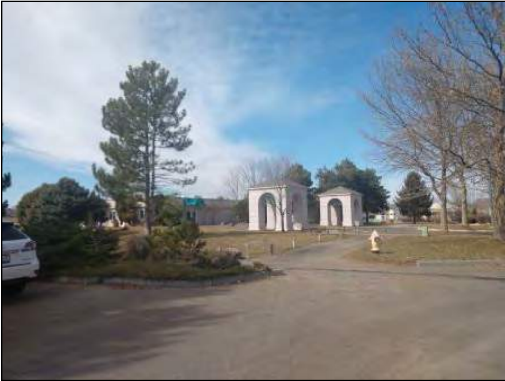
Site looking north
