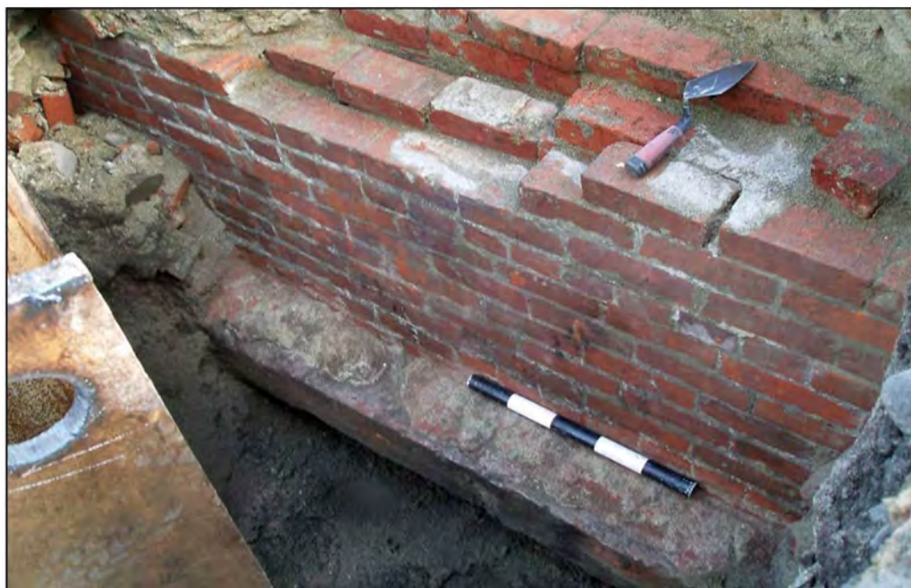
Figure 7. Example of a Buried Brick Foundation
