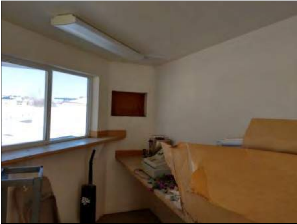
Interior of shack
