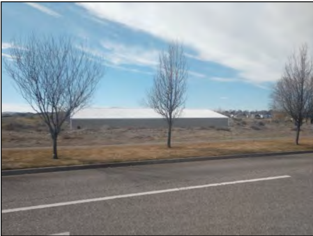
Golf cart shed at the site
