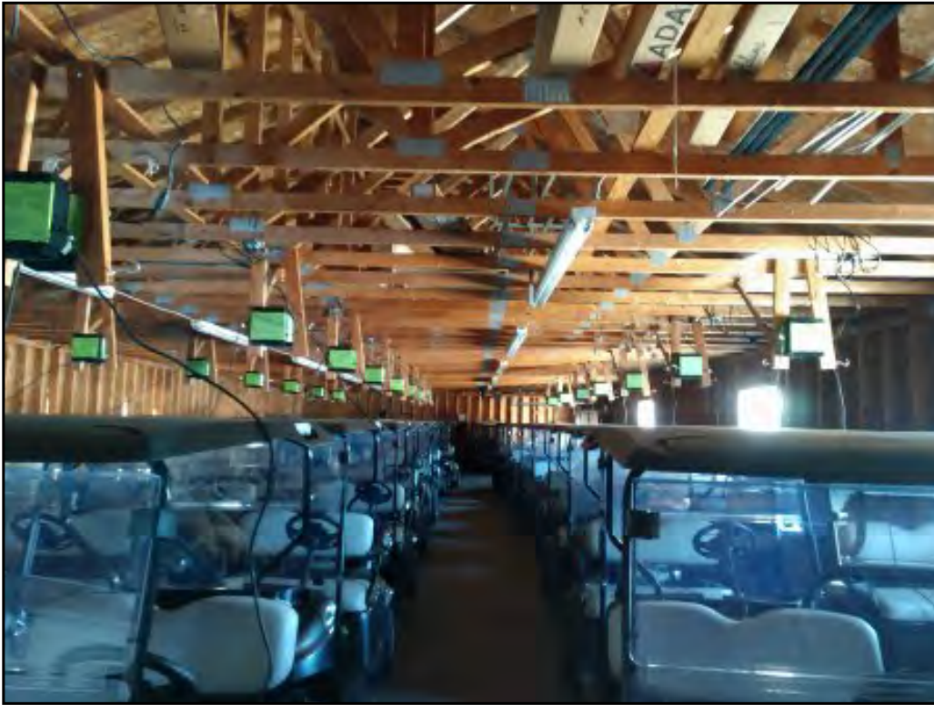
Golf cart shed
