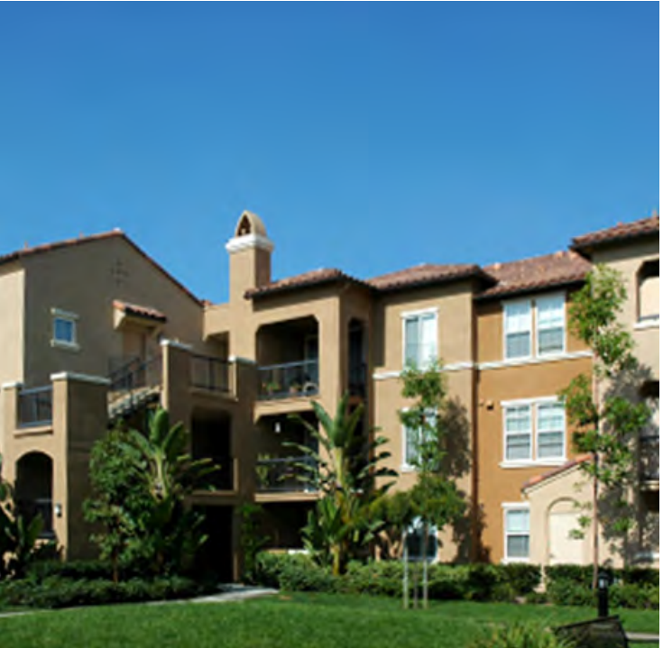
Illustrative Photo: Traditional Walk-up Apartment Building
