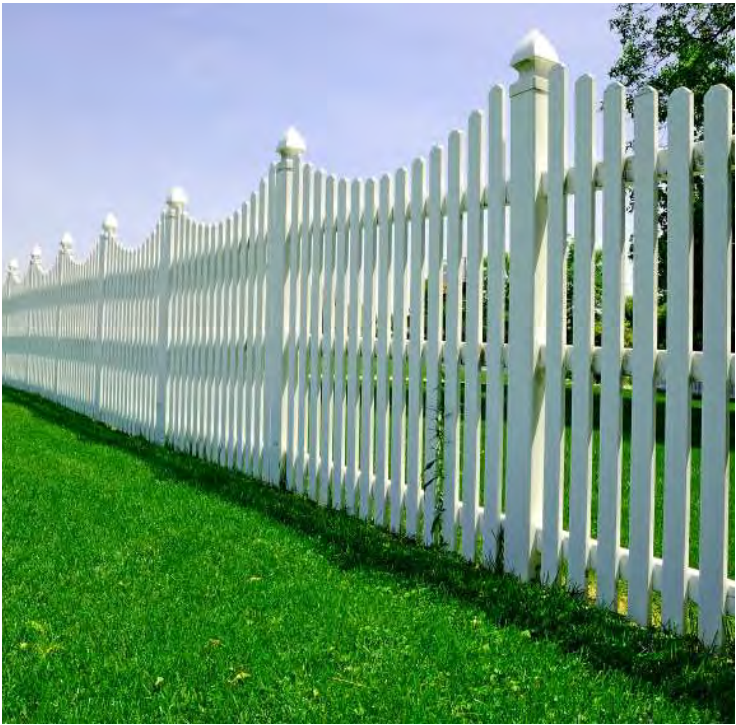
Painted Wood Fencing
