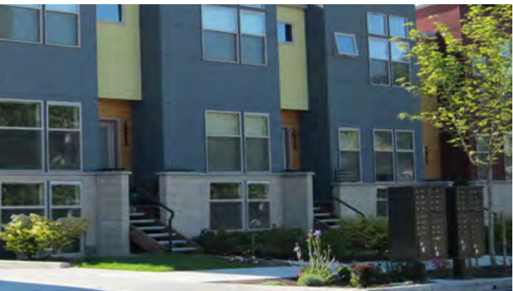
Illustrative Photo: Row House Stoop Frontages
