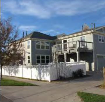
Corner Lot Fencing
