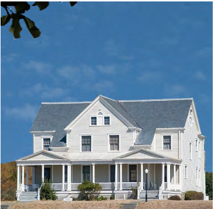
Illustrative Photo: Mid Block Mansion Apartment (4 units max.)
