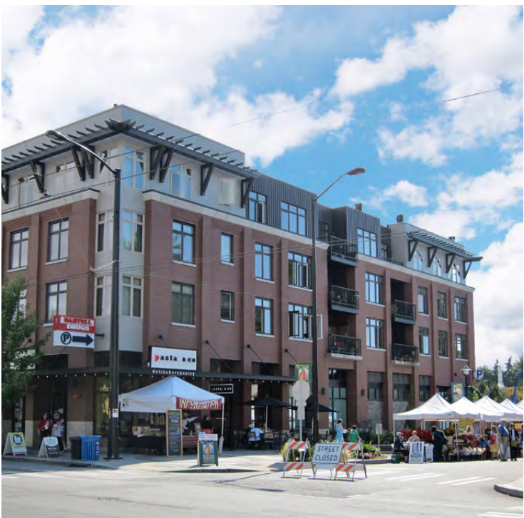
Illustrative Photo: Residential Units above Retail Frontage
