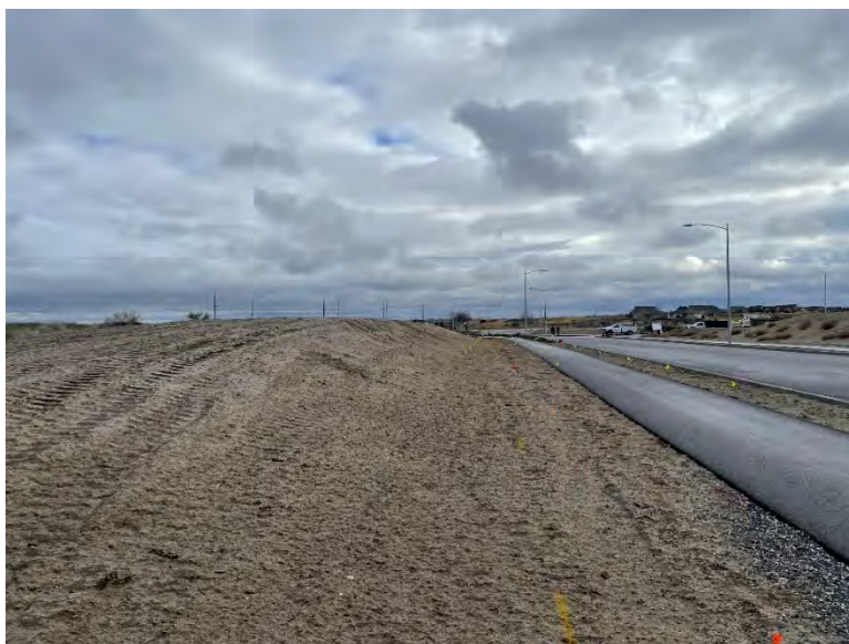
Figure 9. Overview of sidewalk, utilities, and road immediately adjacent to APE; View: E
