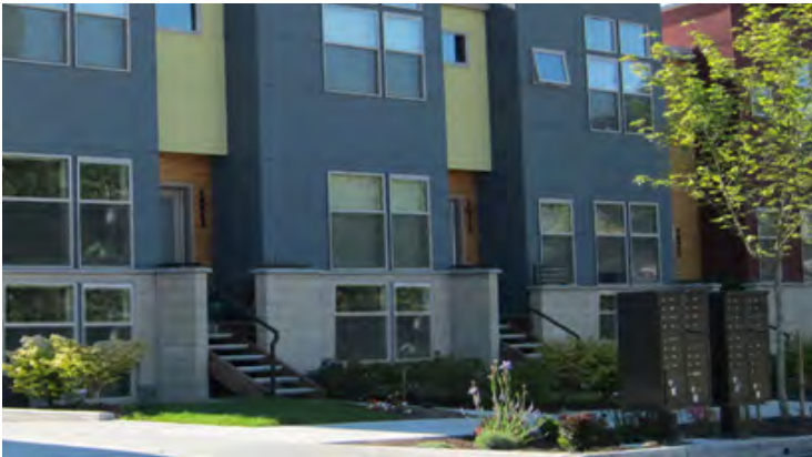
Illustrative Photo: Row House Stoop Frontages
