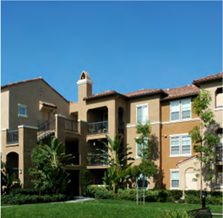
Illustrative Photo: Traditional Walk-up Apartment Building
