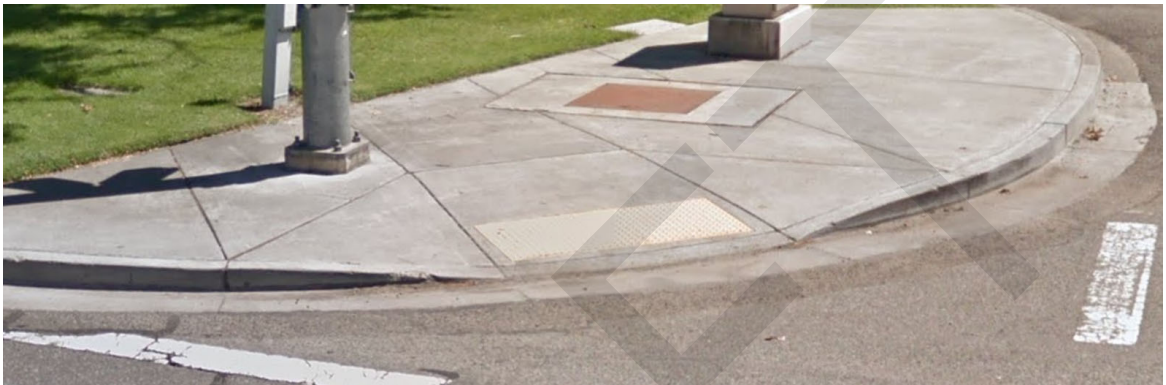
Figure 2- 4 - Example of Diagonal Ramp
