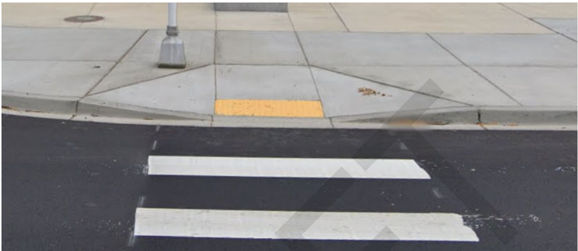
Figure 2-2 - Example of Perpendicular Ramp
