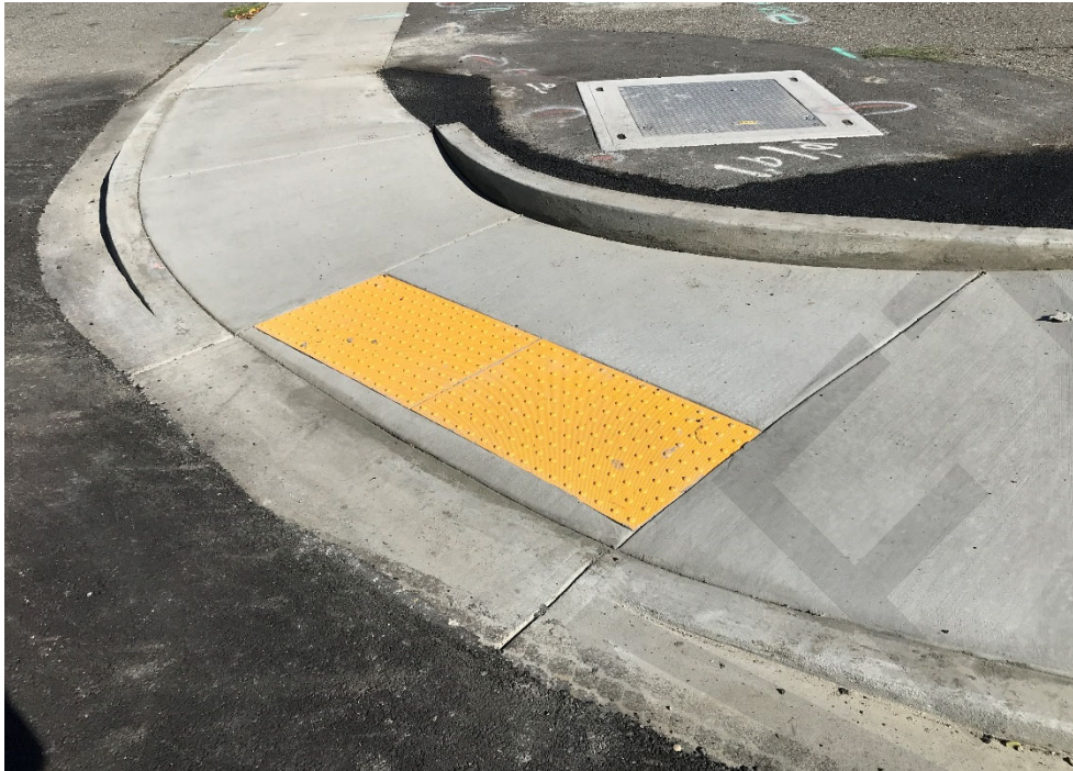
Figure 2-6 - Detectable warning surface
