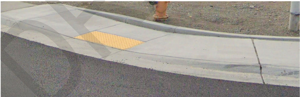
Figure 2-3 - Example of Parallel Ramp
