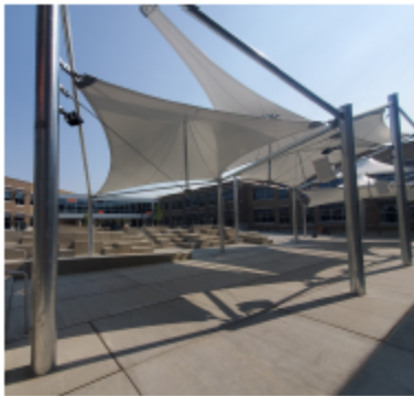
SHADE SAILS AT KENNEWICK HIGH SCHOOL
