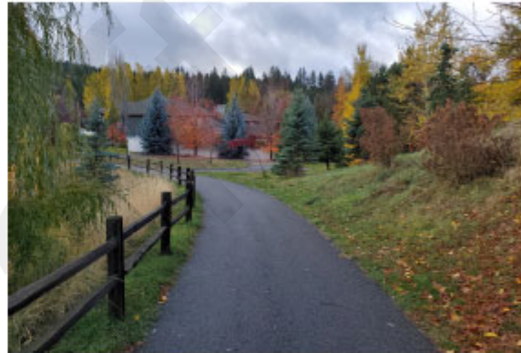
BROWNE MOUNTAIN STORMWATER FACILITY, SPOKANE COUNTY
