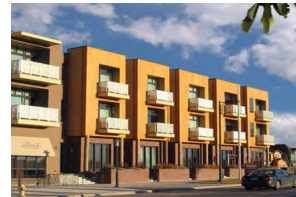
Live/Work Building (8G)
