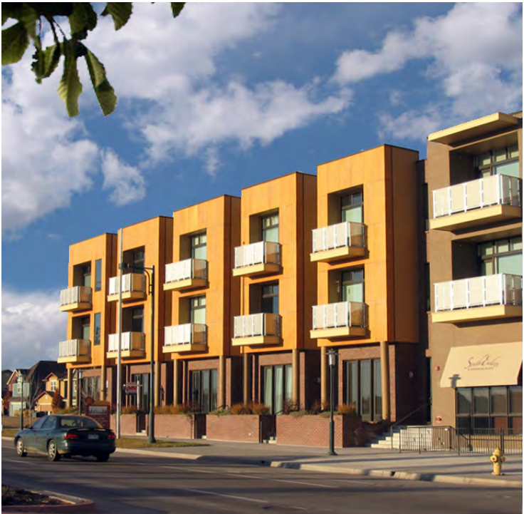
Illustrative Photo: Urban Character Live/Work Building
