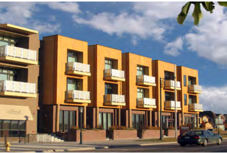
Live/Work Building (8G)
