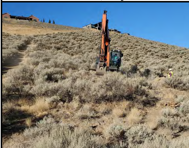
Excavation of test pit TP-1, view looking northwest
