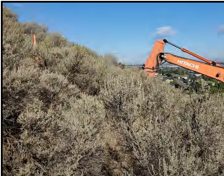
View of surface conditions near test pit TP-3
