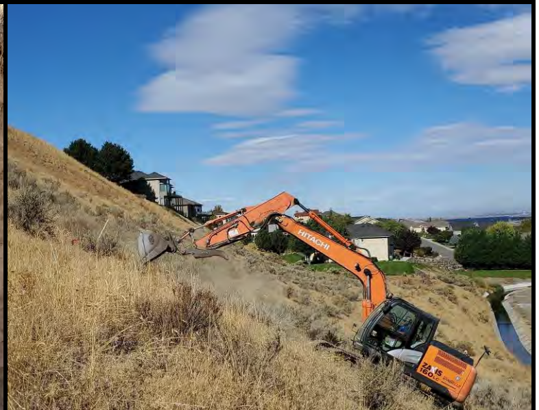
Excavation of test pit TP-5, view looking northwest
