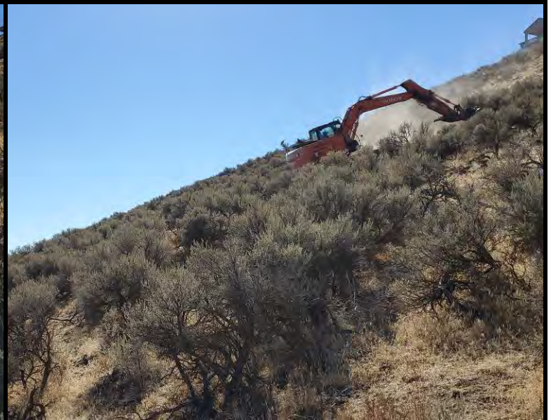
Excavation of test pit TP-4
