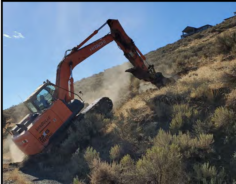
Mobilization to test pit TP-4, view looking south
