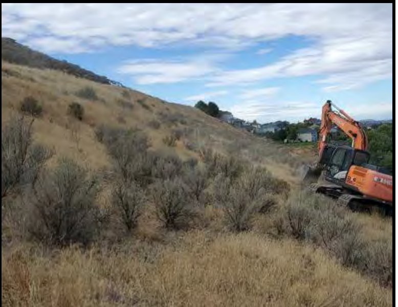
Excavation of test pit TP-8, view looking northwest
