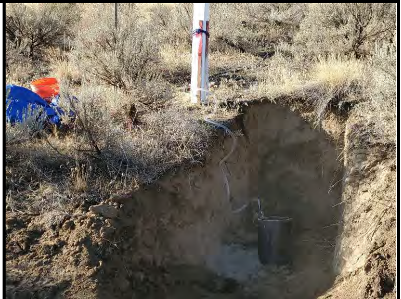
Infiltration test setup at IT-1
