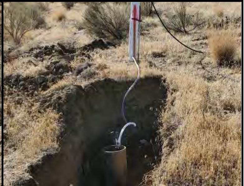
Infiltration test setup at IT-6
