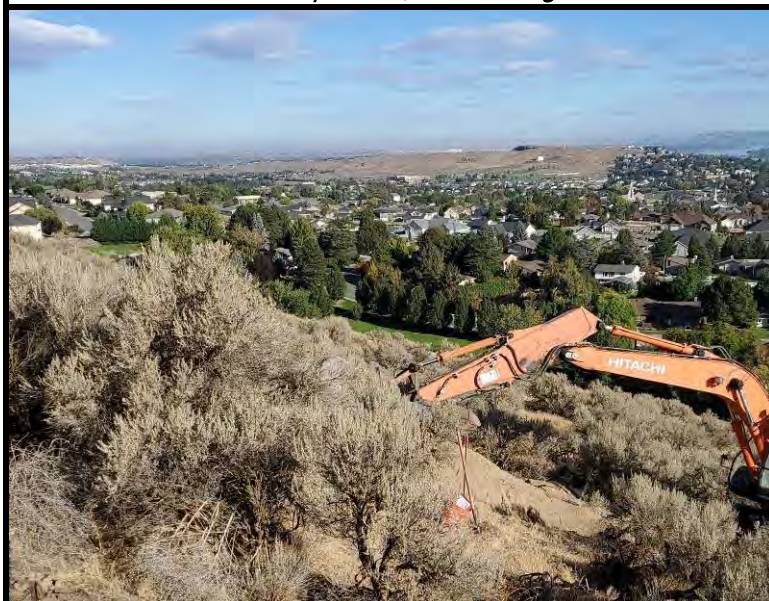
Excavation of test pit TP-2, view looking northeast
