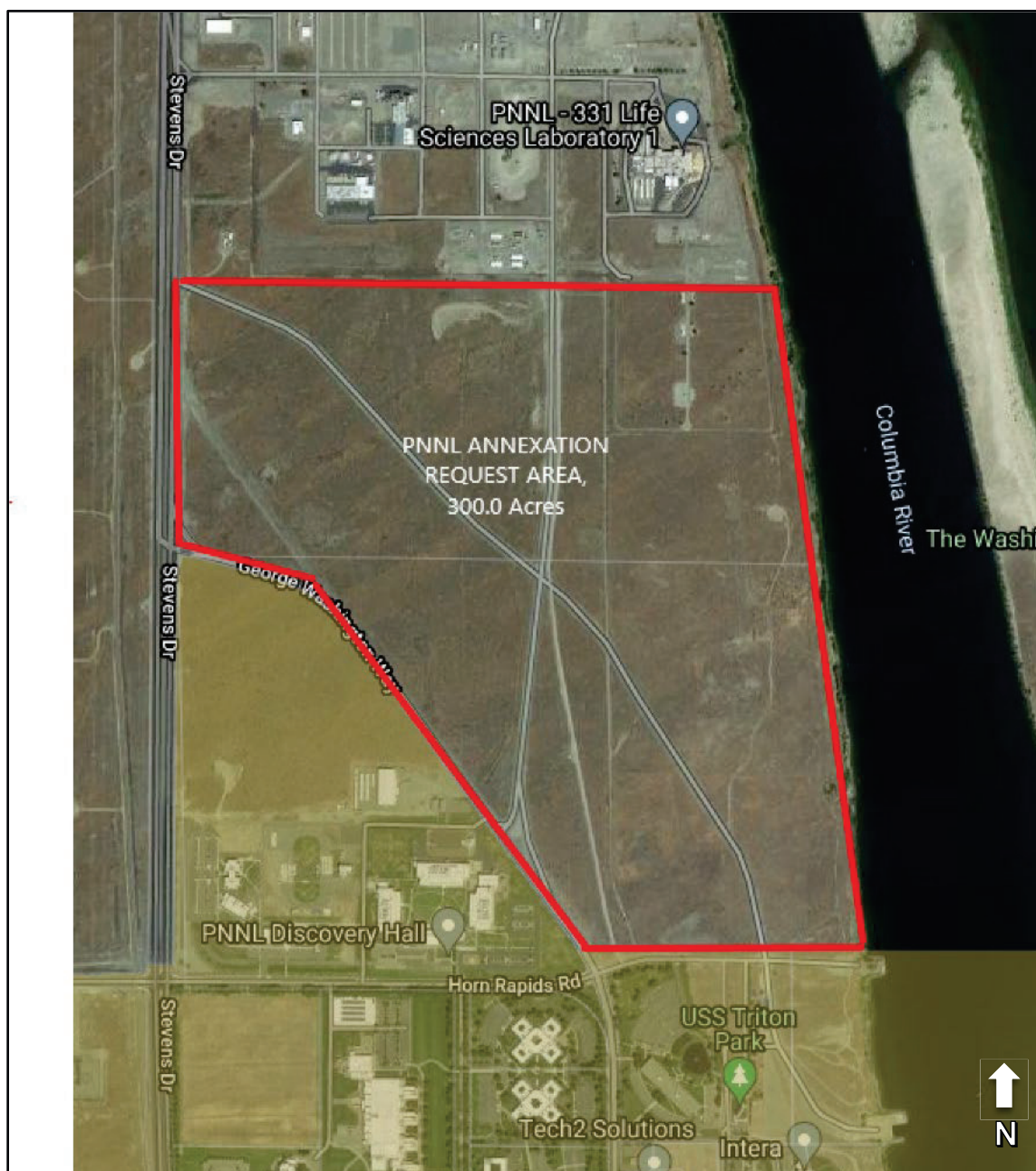
EXHIBIT 1B – Overall Annexation Area Aerial Photo
